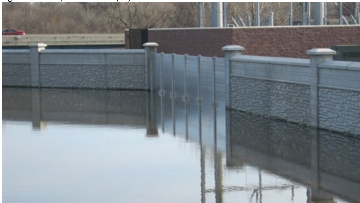
Figure 24. Example of floodwall project in Moorhead
