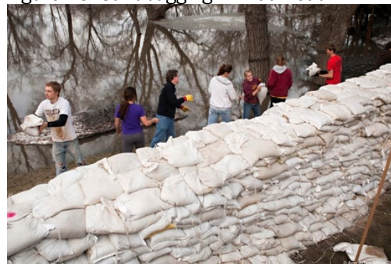
Figure 23. Sandbagging in Moorhead
